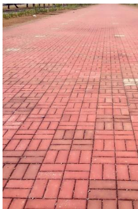
a) Pavement Road
